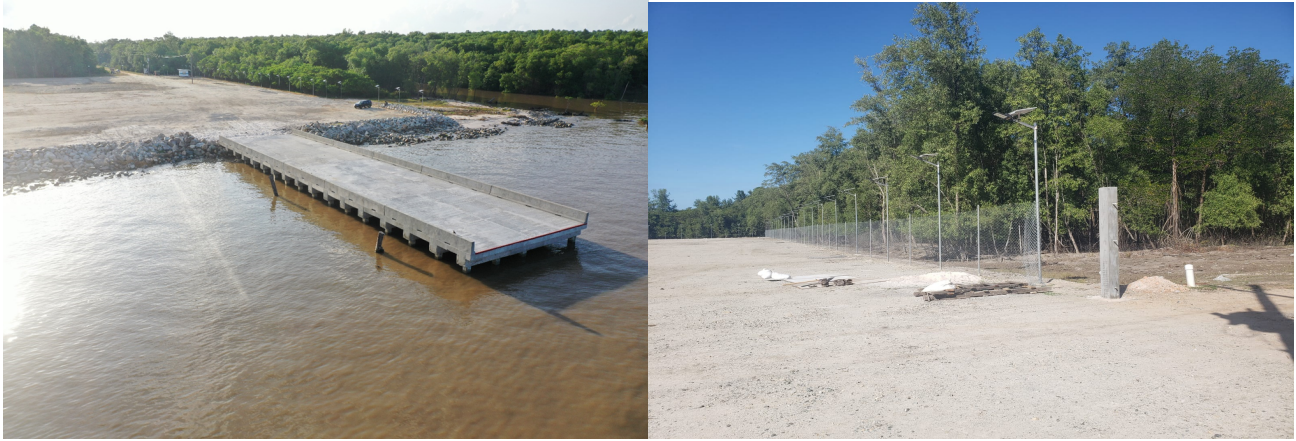
Images: Trestle / Fence installation
