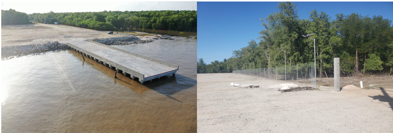
Images: Trestle / Fence installation
