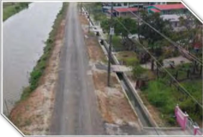
The First **200 meters** of the access road, adjacent to the Seawell village residents, was fully paved with the construction of a **concrete drain** and **concrete bridges** for each resident. The contract for Access Road was amended to include this component.
