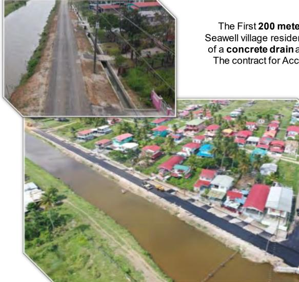
The First **200 meters** of the access road, adjacent to the Seawell village residents, was fully paved with the construction of a **concrete drain** and **concrete bridges** for each resident. The contract for Access Road was amended to include this component.
