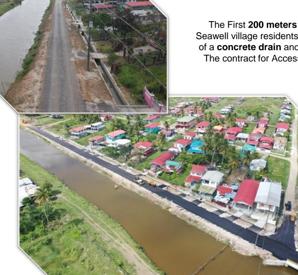
The First **200 meters** of the access road, adjacent to the Seawell village residents, was fully paved with the construction of a **concrete drain** and **concrete bridges** for each resident. The contract for Access Road was amended to include this component.
